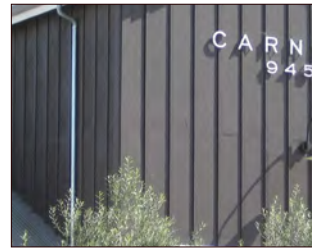
Wood: board and batten
