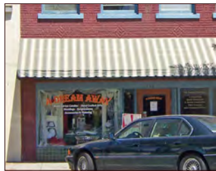
Awning shading at storefront
