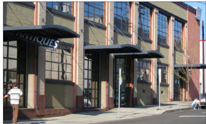
Shed Building type with multiple businesses and their entries from the street.
