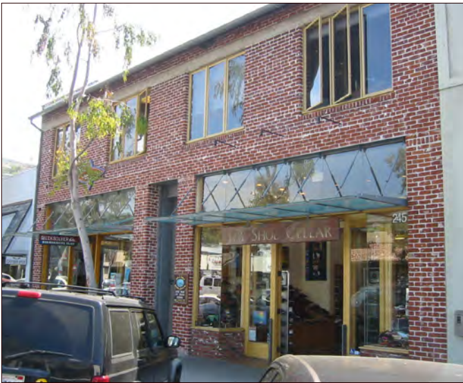
Example: Main Street Commercial style building in brick with clerestory over glass canopies, stores on the ground floor, living units on upper floor.
