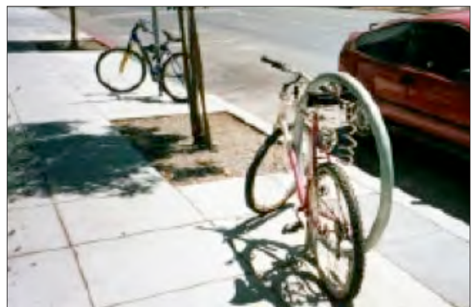
Figure 3.16 Example of an “O” Style Bike Rack Installed on the Sidewalk
