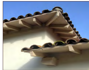
Roof overhang, wooden eave with exposed rafters
