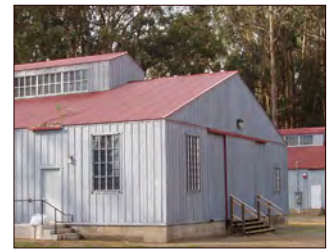
Metal roofs, monitors
