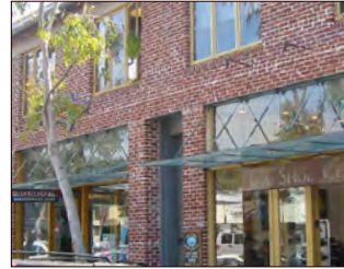
Simple wall plane of brick
