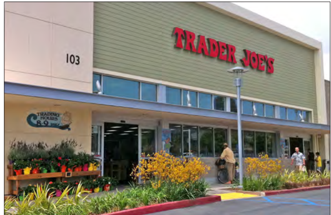
Highway-oriented retail is in buildings with part of their frontage at or near the sidewalk and the other portion fronting parking. Pedestrian access is enhanced by clear delineation of streetscapes that define the building's frontages on the street and parking.
