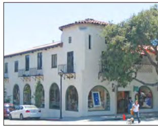
Single volume, corner tower
