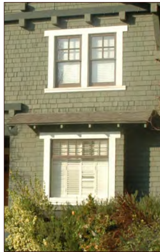
Openings are stacked with the same area being used for either one or two windows. Note the simple shed awning over the ground floor window.
