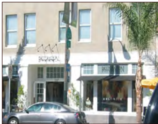
Storefront with double hung windows above
