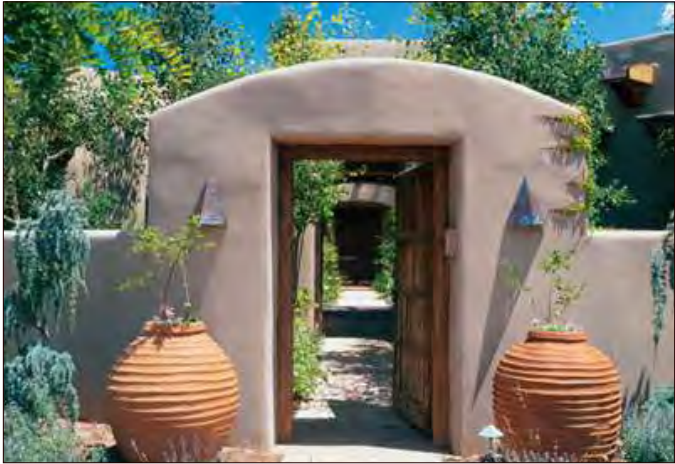
Walled Yard Example - The walled yard frontage enables open areas along front or side lot lines to be partially enclosed while defining the streetscape in a complementary manner.
