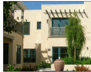
Simple plaster plane, no base
