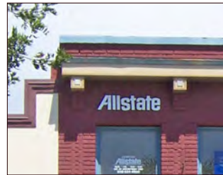
Parapet and bracketed cornice
