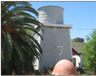
Water tank, bread oven
