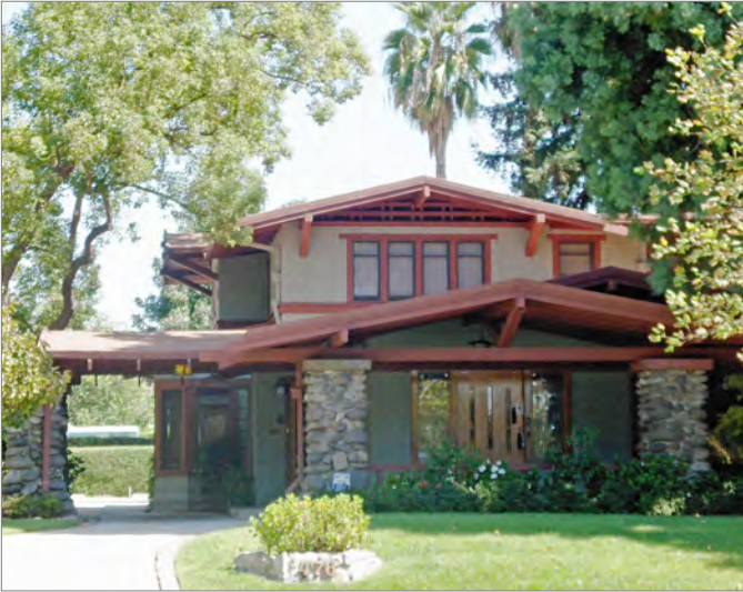
Example: Craftsman bungalow with deep set porches, exposed rafter tails and beams, masonry pier/foundation.
