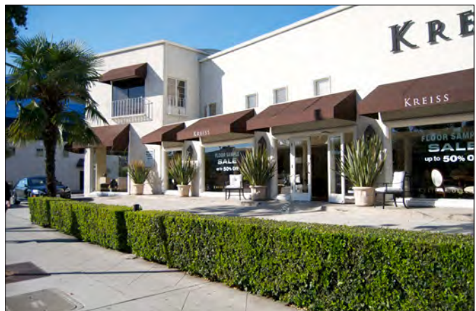
Parking Courts provide convenient parking while maintaining a strong relationship with the streetscape.
