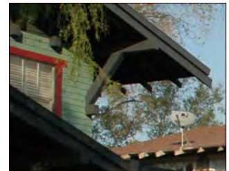
Deep overhangs to emphasize horizontality and to provide shade.
