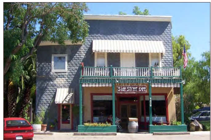
Gallery Example - a 1 story version with colonnade, roof, and open deck which shades both the sidewalk and storefront display windows.
