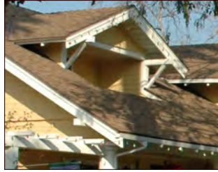
Roof braces are typically large and emphasize their structural role and qualities
