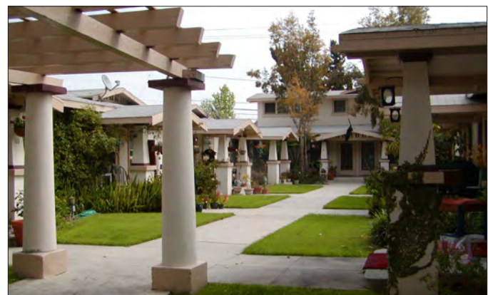
Bungalow Court Building type with some multiple-story buildings.
