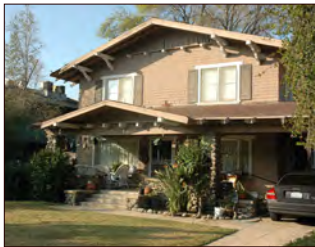
Simple, large planes highlighted by gables facing the street
