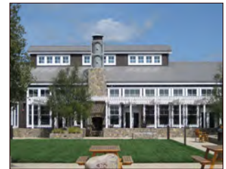
Monitors on roof ridge.
