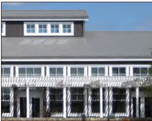
Clerestory windows, & regular patterns of window placement relate to structure
